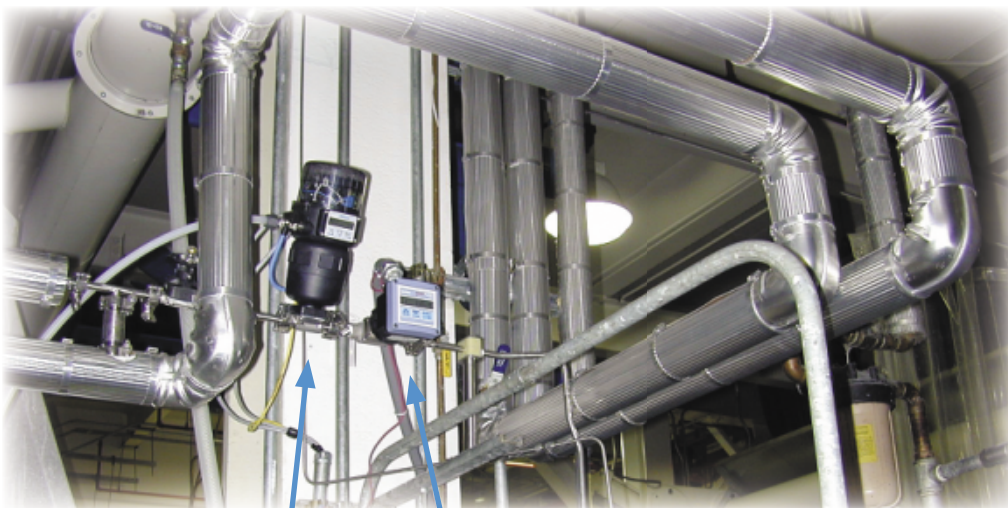
Type 2031 Diaphragm with PID TOP Control
